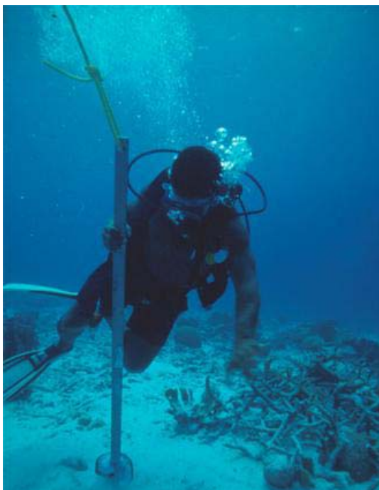
Fig 13. A marine park ranger installs a mooring buoy which will reduce anchor damage to corals in Bonaire Marine Park (Netherlands Antilles) Photo: Dee Scarr
